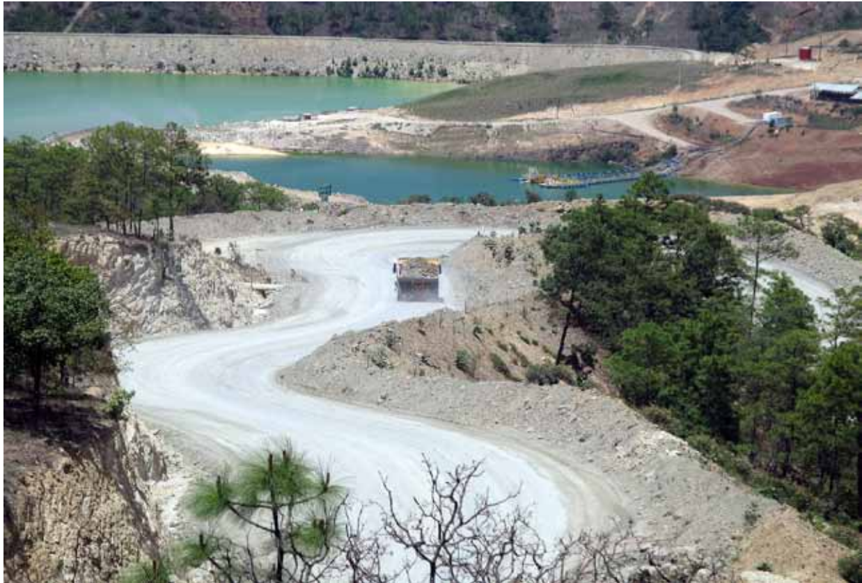
A lake of toxic industrial waste has formed on the valley floor. It includes cyanide, used in the extraction of gold from the mine, which is thought to have polluted the groundwater. → D.B.
